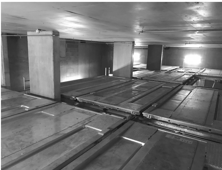
Completed puzzle installation ready for use by tenants
