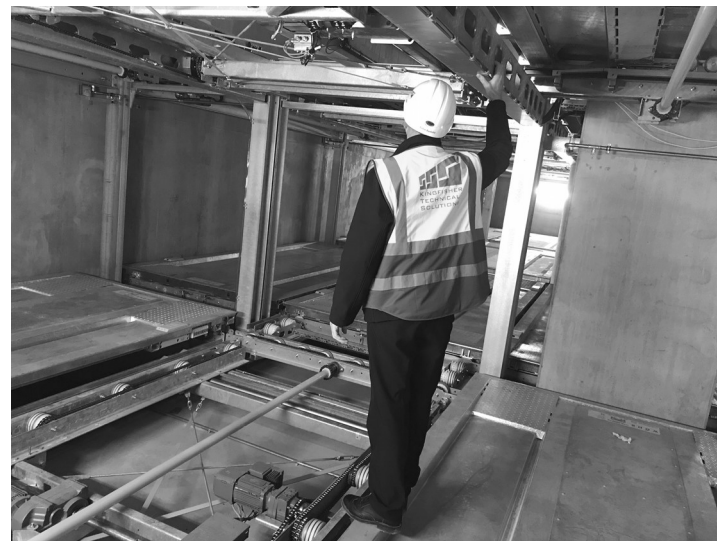
Final inspection of puzzle system prior to handover
